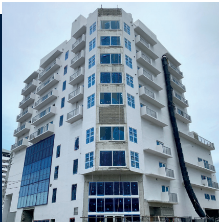
EAST RIVER LIVING - WEST BRICKELL
